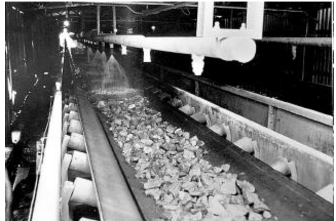
Fig. 4.7.1(b)—Cooling coarse aggregate by chilled water spray and inundation
