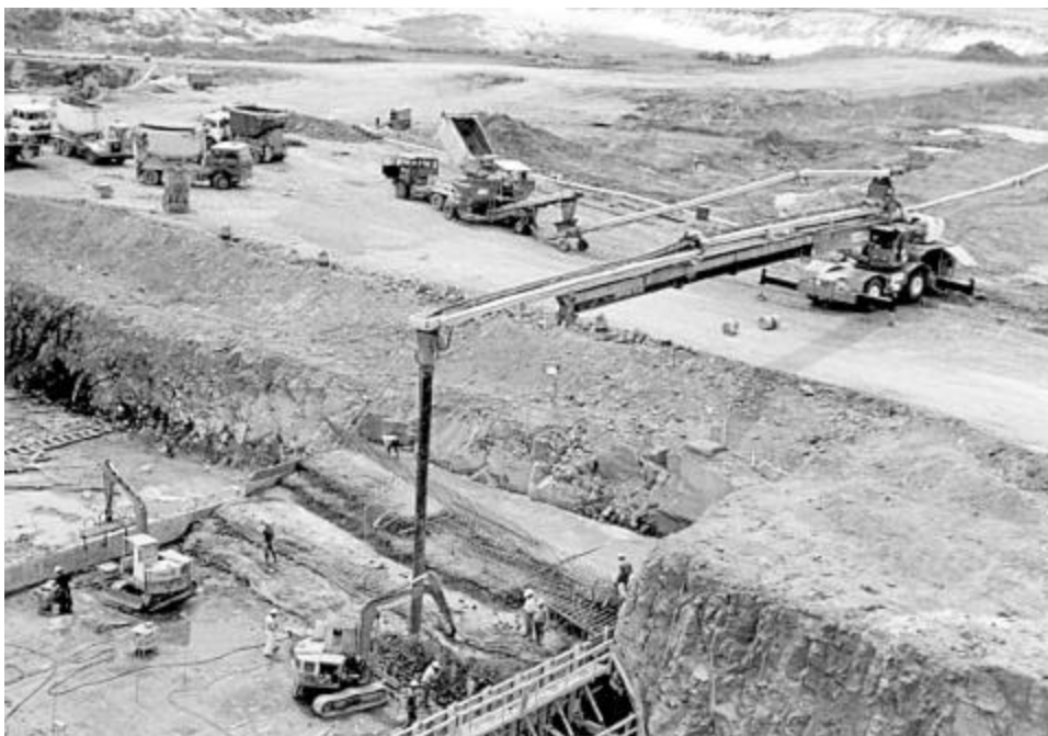
Fig. 4.3.7—Placement of mass concrete by conveyor belt
