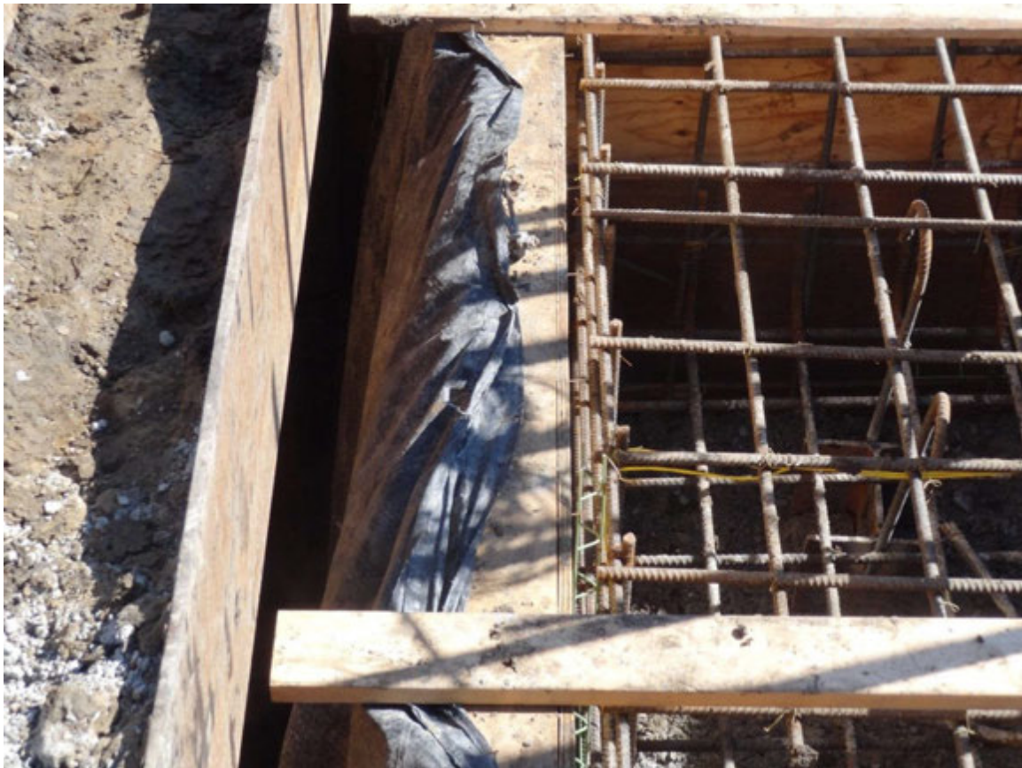
Figure 5.10 Insulation attached to wood formed footings
