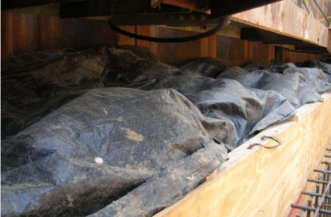
Figure 5.12 Shored formwork insulating blanket
