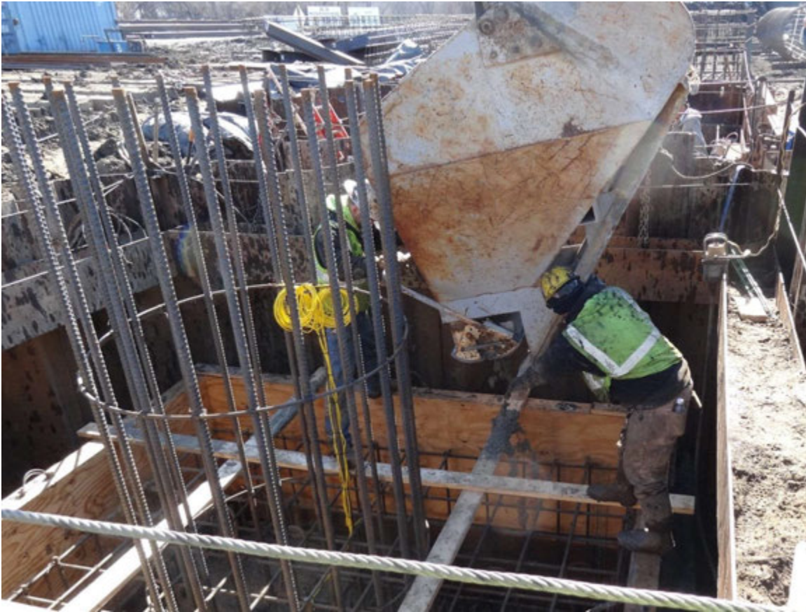
Figure 5.8 US 34 Bridge Pier 2 footing concrete placement
