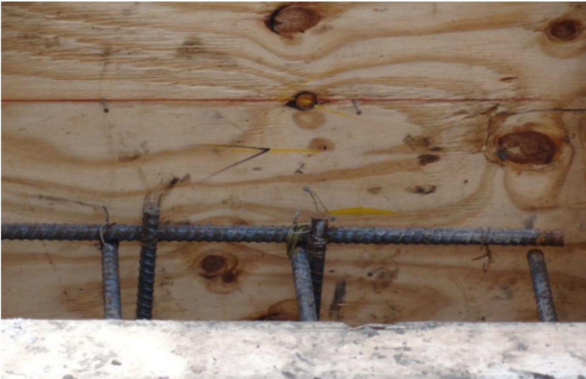
Figure 5.23 Typical rebar cover for mass concrete footing
