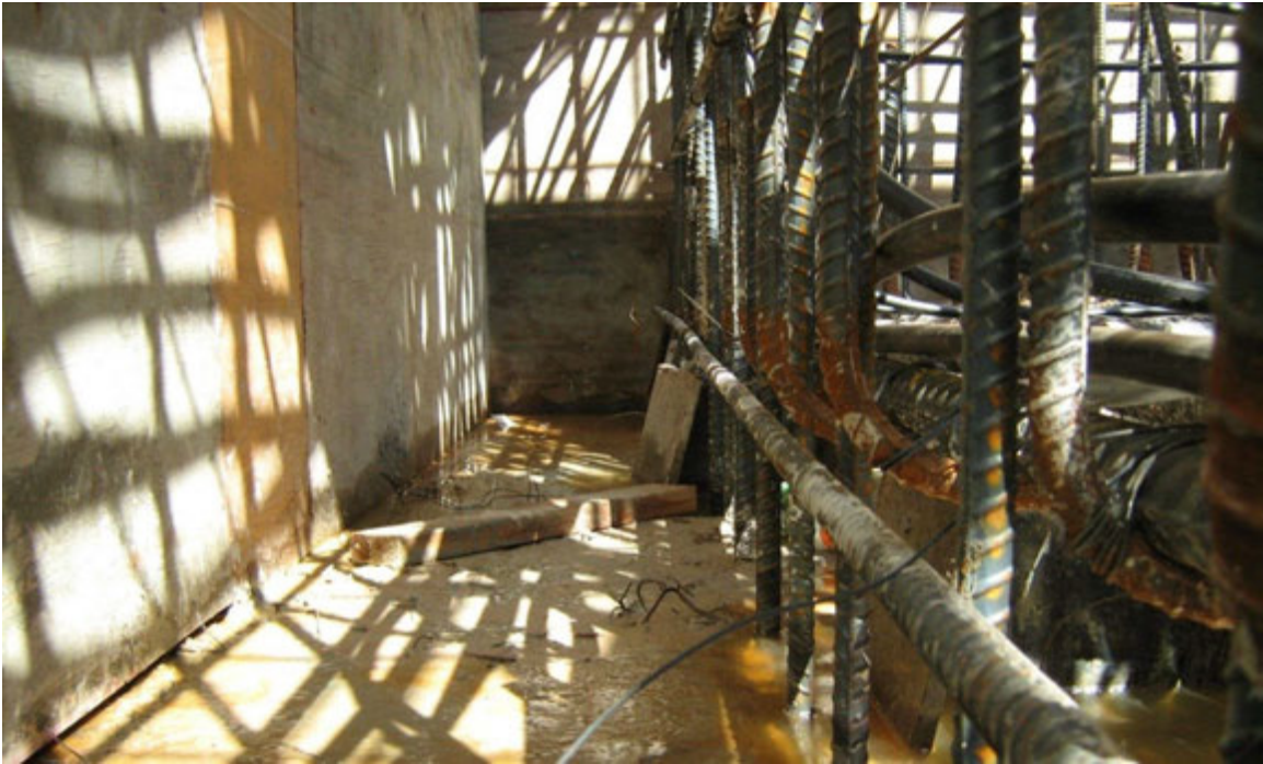
Figure 5.21 Distance between formwork and outermost rebar/thermal sensor location – large distance
