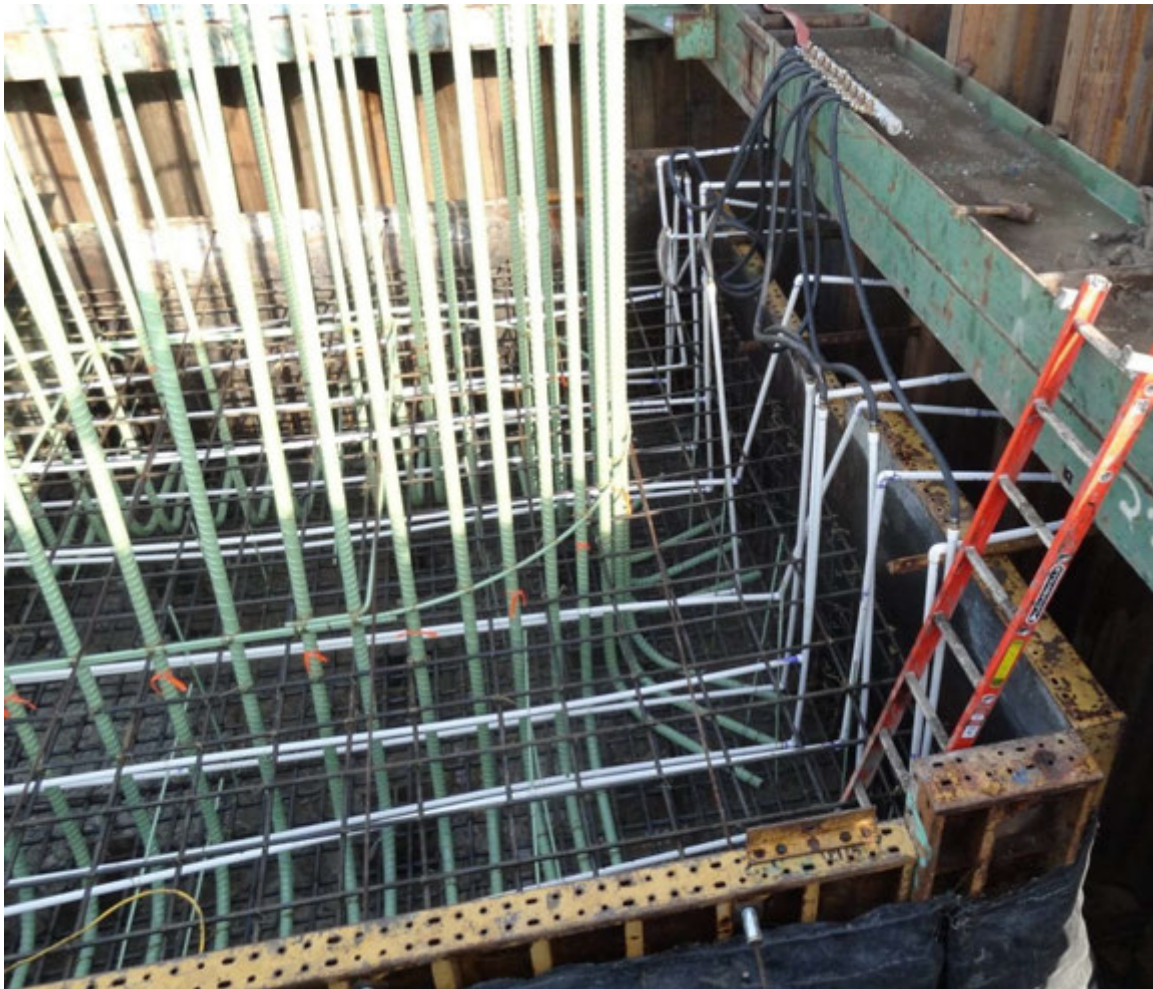
Figure 5.20 Installed PVC piping on US 34 Bridge footing
