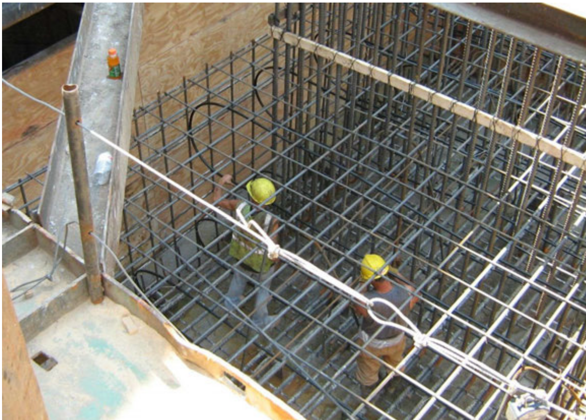
Figure 5.19 PEX cooling pipes being installed on a WB I 80 bridge footing
