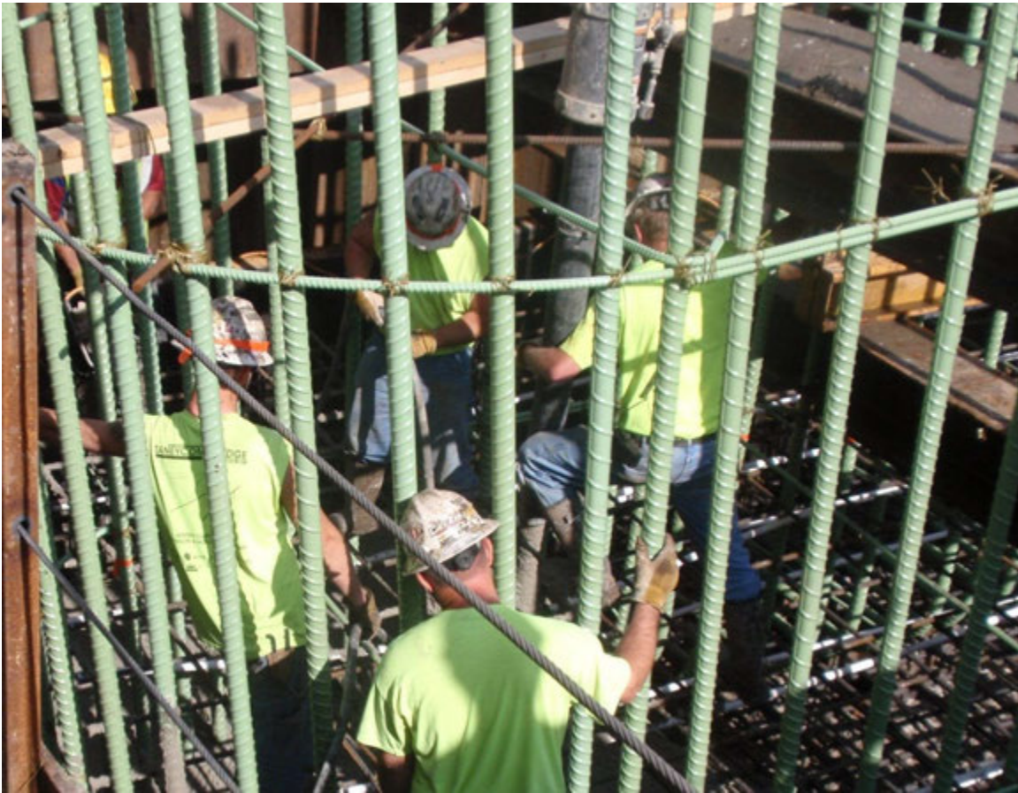
Figure 5.7 US 34 Bridge Pier 4 footing concrete placement
