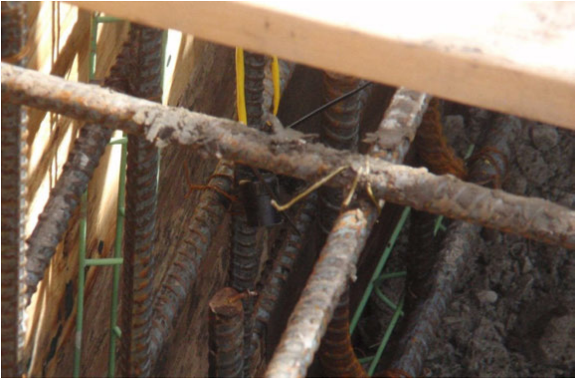
Figure 5.22 Distance between formwork and outermost rebar/thermal sensor location – small distance
