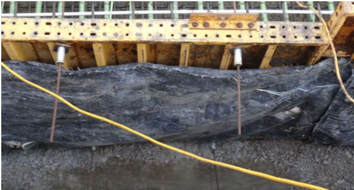
Figure 5.14 Steel formed footing with insulating blanket
