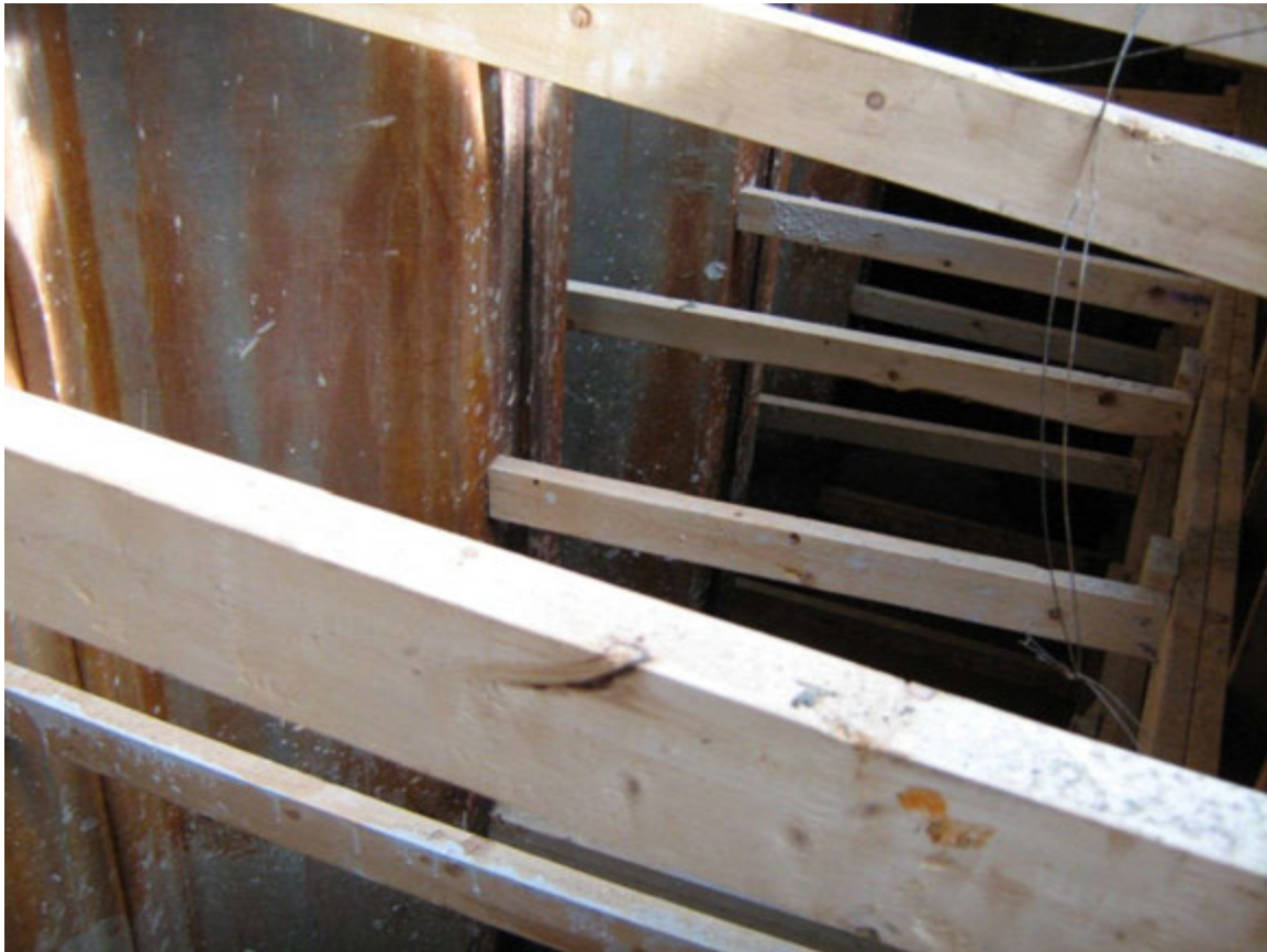
Figure 5.11 WB I-80 Bridge wood formed footing shoring
