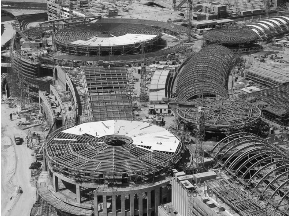
Cladding works Dubai Mall, Dubai, United Arab Emirates
