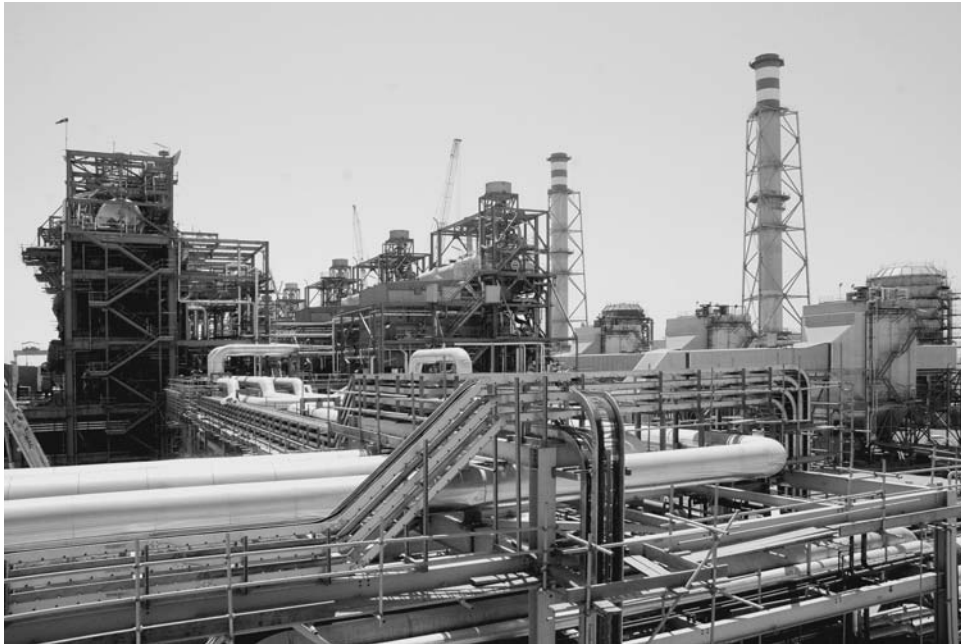
Rabigh Independent Water, Steam, and Power Plant, Rabigh, Saudi Arabia
