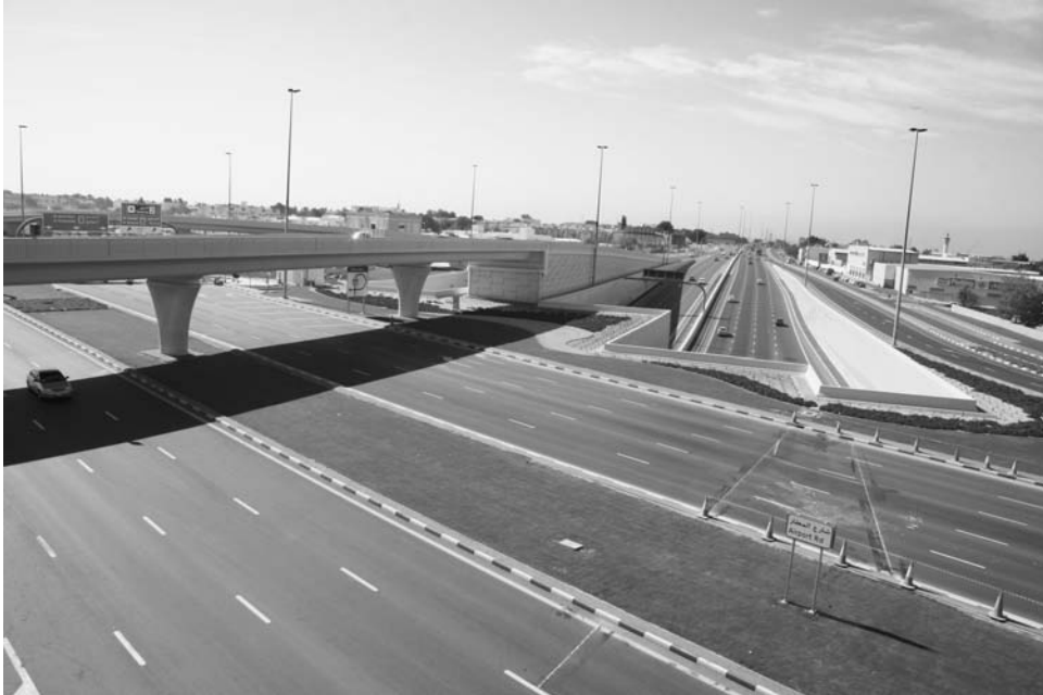
Expansion Nadd Al Hamar/Beirut Roads Tunnel, Dubai, United Arab Emirates
