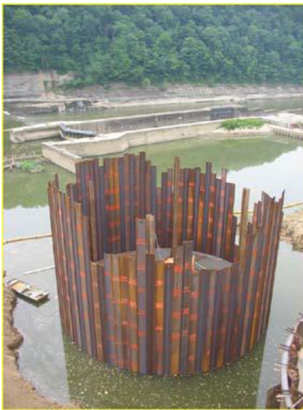
Figure 3: Concrete-filled cellular sheet pile cell
