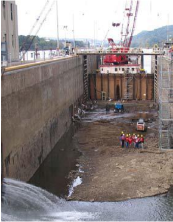
Figure 8: Dewatered chamber at McAlpine
