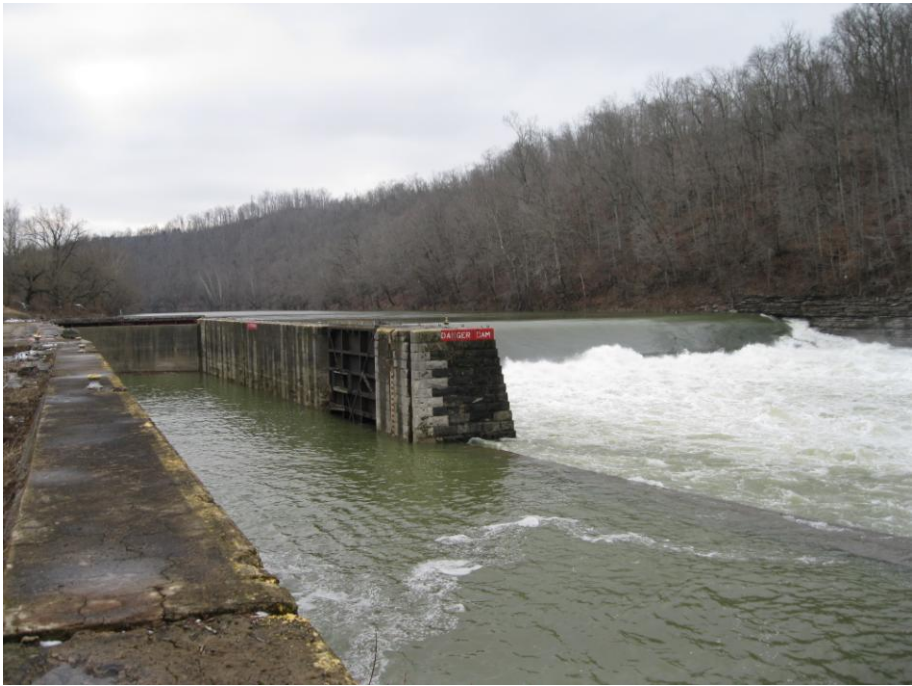
Figure 1: Kentucky River Lock and Dam No. 8
