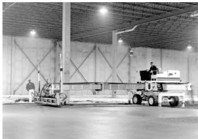
Fig. 8.2.3.2—Laser controlled screed
