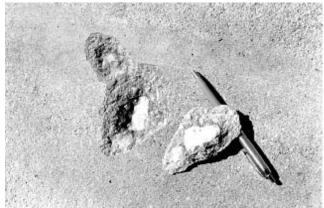
Fig. 11.6—A popout is a small fragment of concrete broken away from the surface of a slab due to internal pressure, leaving a shallow, typically conical, depression
