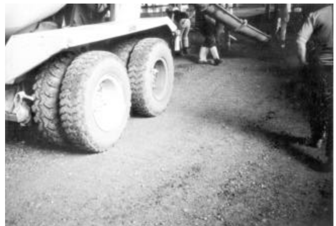
Fig. 4.1.1—Proofrolling by loaded ready mix truck
