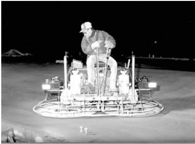
Fig. 8.2.4.4—Double-riding trowel with clip-on pans
