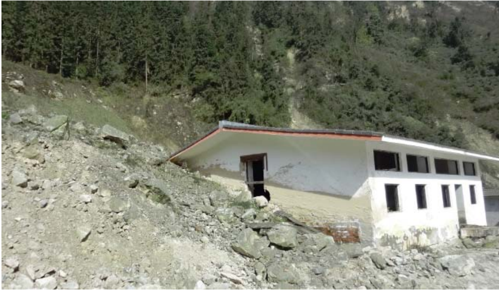
Figure 5.2 Landside damage in Sichuan, China, 2010
