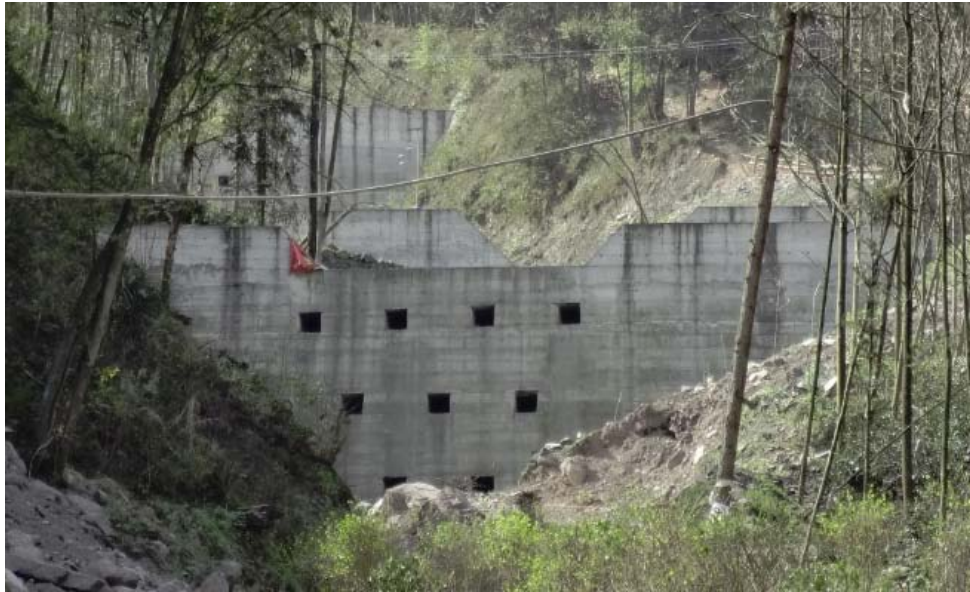
Figure 5.4 Check dam for debris flows
