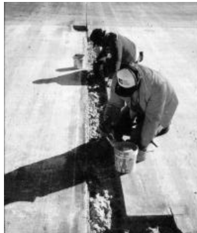
Figure 5.9 Application of bonding agent
