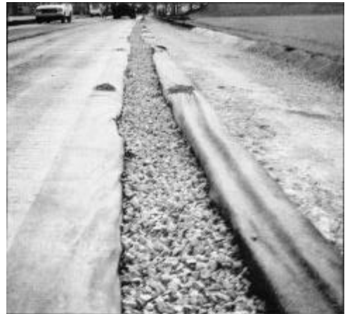
Figure 12.6. Lined trench with coarse backfill
