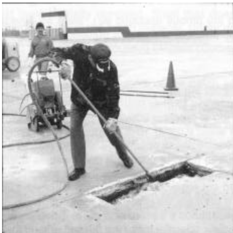
Figure 5.6. Cleaning exposed faces
