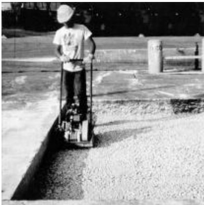
Figure 4.11. Patch area compaction
