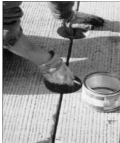
Figure 10.4. Grooving sidewalls
