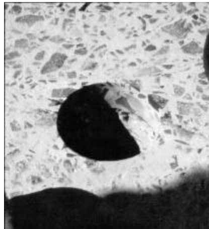
Figure 10.6. Cleaned patch area
