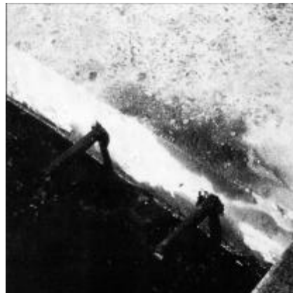
Figure 4.12. Smooth steel dowels
