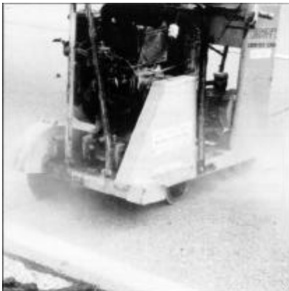
Figure 4.5, Diamond blade sawing
