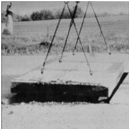
Figure 4.9. Lift-out method
