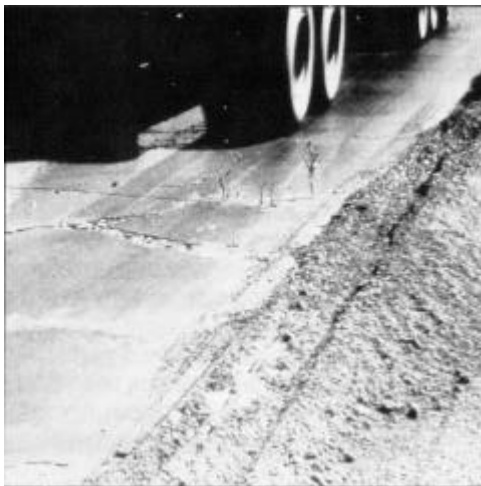
Figure 12.1. Pavement pumping
