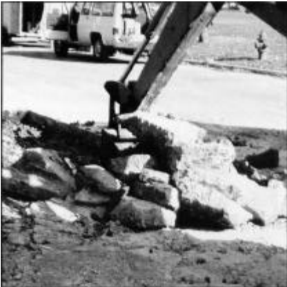
Figure 4.7. Concrete removal
