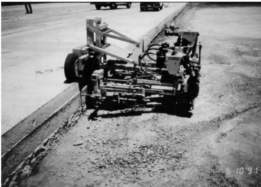
Figure 4.14. Drilling multiple holes
