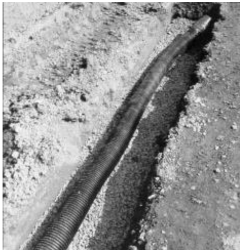
Figure 12.3. Flexible drainage pipe
