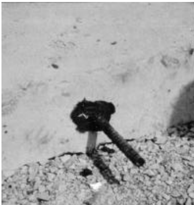
Figure 4.13. Deformed reinforcement
