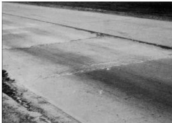
Figure 5.2. Severe spalling
