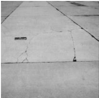
Figure 4.1. Shattered slab
