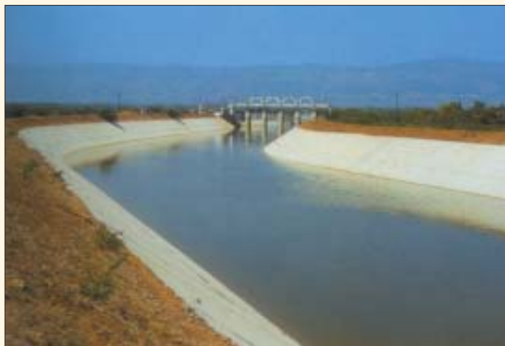
▶ SAI GANGA approach canal for water supply to Chennai Metro.
