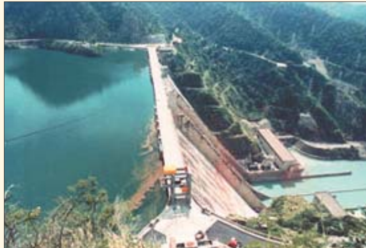
▶ THE BHAKRA DAM is a majestic monument across river Sutlej. The construction of this project was started in the year 1948 and was completed in 1963 . It is 740 ft. high above the deepest foundation as straight concrete dam being more than three times the height of Qutab Minar. Bhakra Dam is the highest Concrete Gravity dam in Asia and Second Highest in the world.
