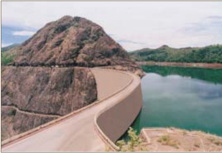
◀ THE IDUKKI HYDROELECTRIC PROJECT, KERALA : The reservoir covers nearly 60 square kilometres and has a catchment of 649 square km. Water from the reservoir is taken down to the underground power house at Moolamattom through an underground tunnel, yielding an average gross head of 2182 feet (665 metres). The project has an installed capacity of 780 MW with firm power potential of 230 MW at 100 per cent load factor.
