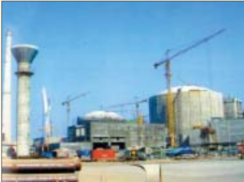
TARAPUR ATOMIC POWER PROJECT : Reactor Building no. 3 & 4.
