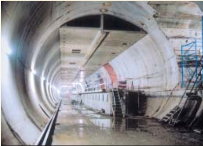
◀ DELHI METRO Railway Station under construction.
