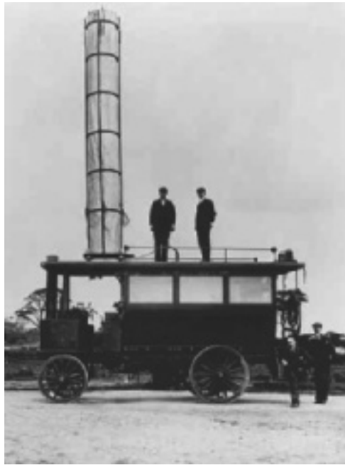
Figure 8.18 An early mobile transceiver: the antenna is located on the roof of the bus. (Reproduced by permission of © 2001–2004 Marconi Corporation plc)
