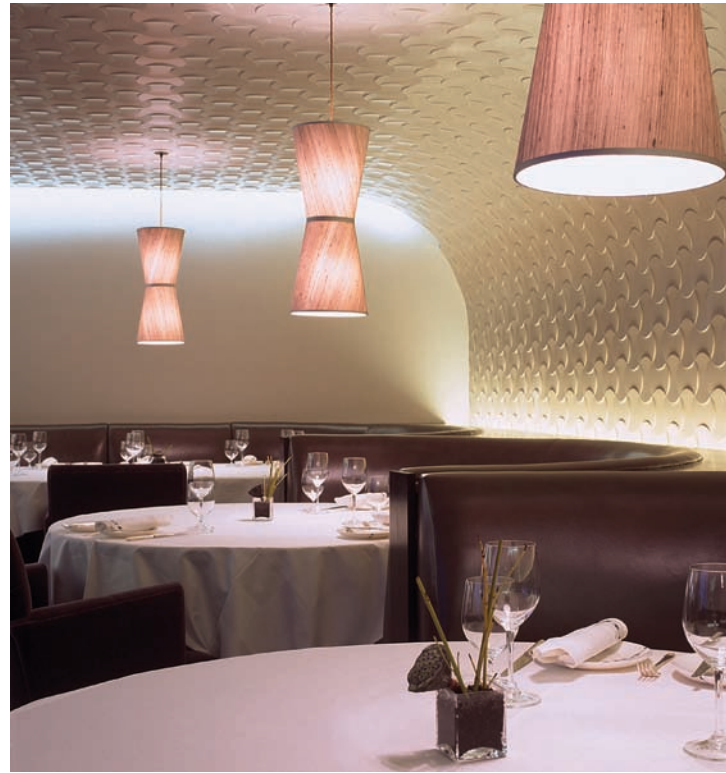
These decorative plaster tiles by Robin Ellis Design for Butcher Plasterworks, seen here in a restaurant designed by Claire Nelson, create a non-uniform surface that has positive acoustic qualities, as well as great decorative potential. The elimination of hard, flat surfaces helps reduce the reflection of unwanted sound waves.
