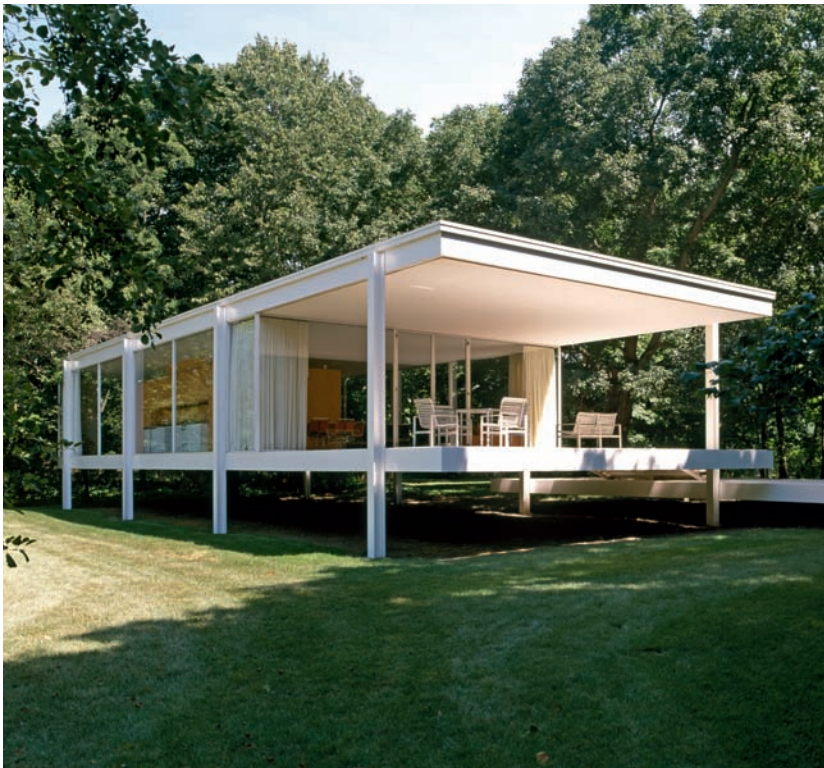
The framed structure of The Farnsworth House by Mies van der Rohe in Plano, USA, is clearly evident and is a major visual feature of this iconic design. It is considered by many to be one of the most beautiful buildings ever designed.
