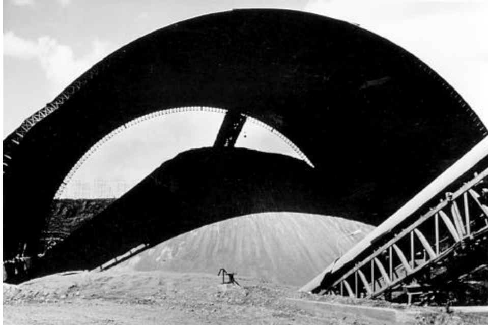
Fig. 4.7.1(a)—Metal cover over drained fine aggregate stock pile to reduce heat absorption
