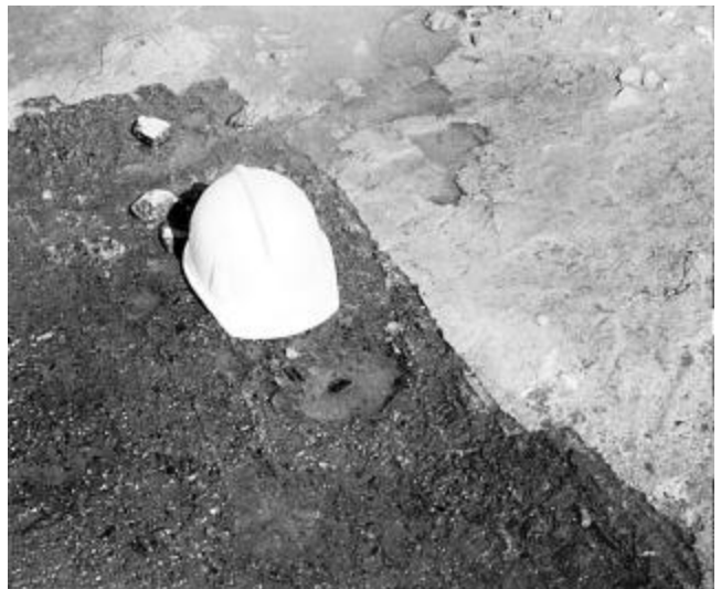
(b) High-pressure water-blast treatment
