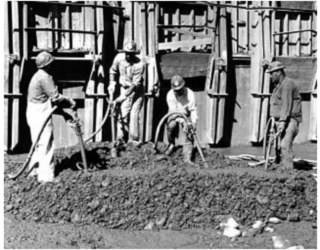
Fig. 4.3.10—Consolidation of low slump mass concrete placed by bucket
