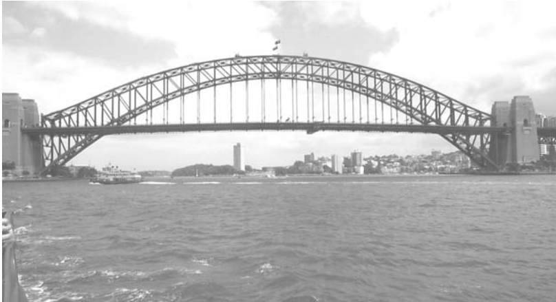
Figure 1.1 Sydney Harbour bridge.
