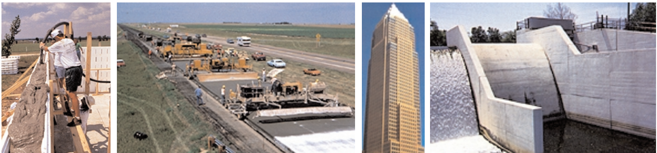
Fig. 3-4. Fly ash, slag, and calcined clay or calcined shale are used in general purpose construction, such as (left to right) walls for residential buildings, pavements, high-rise towers, and dams. (67279, 48177, 69554, 69555)
