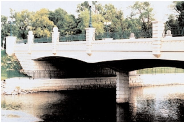
Fig. 3-9. Although they can be used in general construction, silica fume and metakaolin are often used in applications such as (left) bridges and (right) parking garages to minimize chloride penetration into concrete. (68681, 69542)
