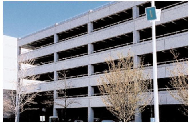
Fig. 3-9. Although they can be used in general construction, silica fume and metakaolin are often used in applications such as (left) bridges and (right) parking garages to minimize chloride penetration into concrete. (68681, 69542)
