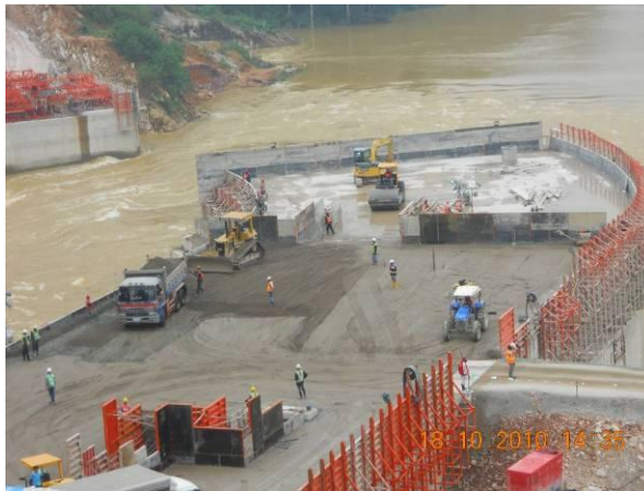
Figure 12 RCC production continues during overtopping event
