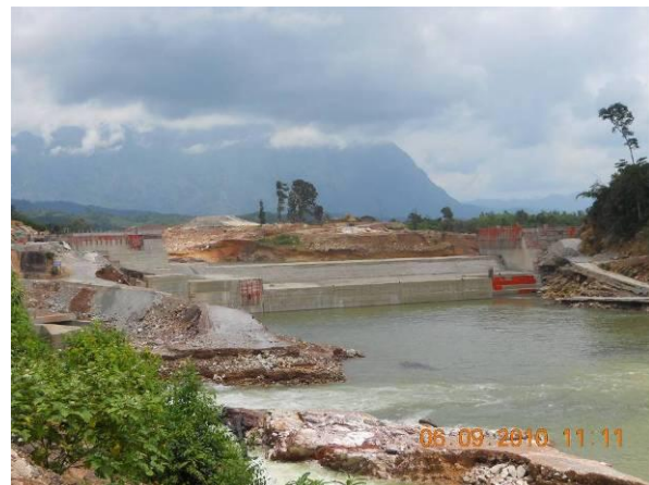
Figure 9 RCC integrated spillway after river receded No damage to RCC structure
