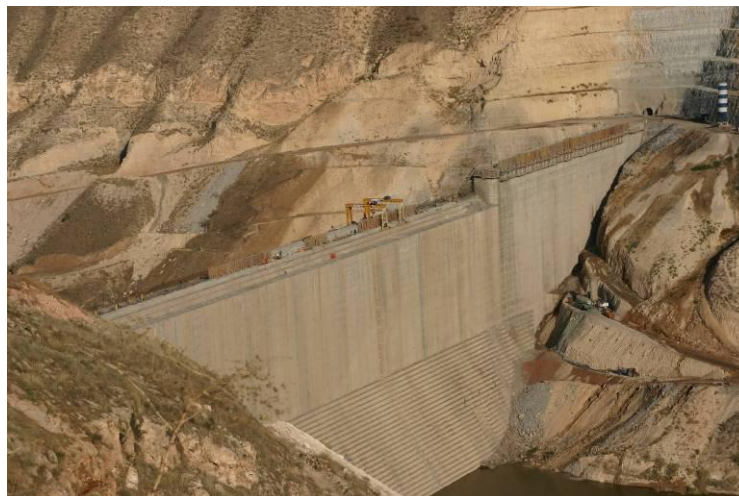
Figure 3 Al Wehdah RCC dam Jordan
