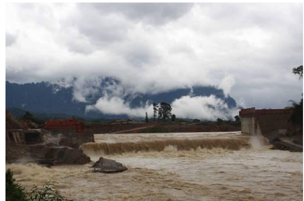
Figure 11 Nam Gnaoung Dam third overtopping 3,000 m 3 /sec over dam
