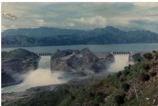
Figure 1 Tarbela earthfill dam
