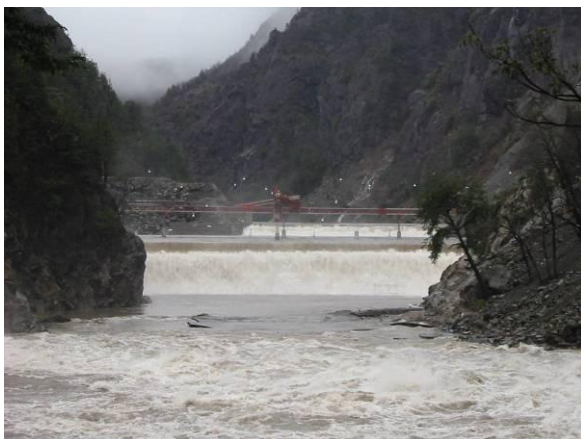
Figure 5 Second overtopping event 155 m tall Ralco dam (Chile)
