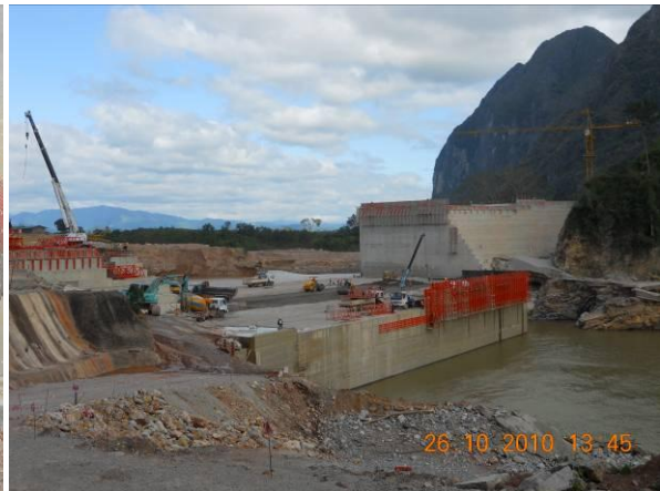
Figure 13 Nam Gnoang dam after third flood RCC resumed
