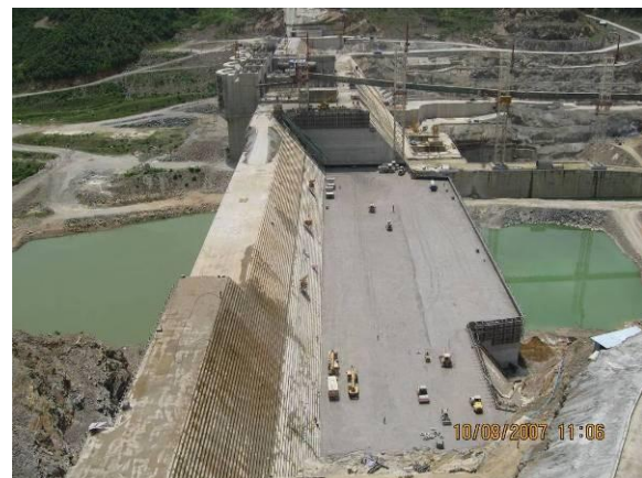
Figure 6 134 m tall Yeywa RCC dam (Myanmar)
