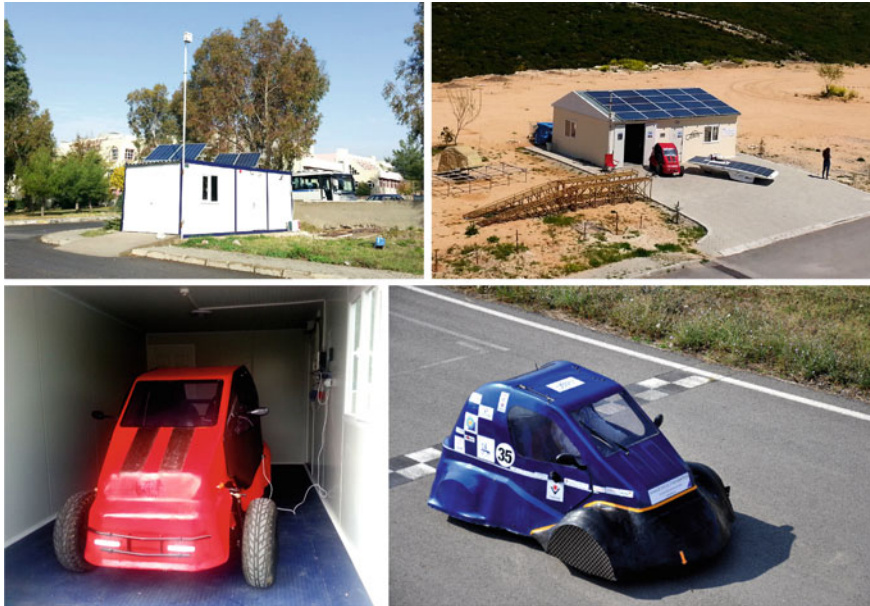
Fig. 11.24 A Charging stations (DECharge 1, 2 and 3) in campus area and charging EVs (DEMobils) at the station
