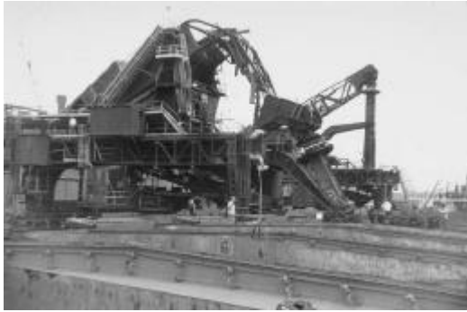
Figure 3. Crane failures resulting from crack growth
