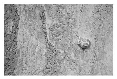
Plate 15b. Sand runs on a concrete wall surface
