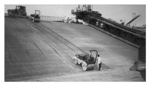
**Plate 4a.** Rollers compacting side slopes of power channel; filter layers and concrete to follow. Ghazi Barotha Hydropower project, Pakistan 1999
