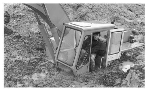
**Plate 5b.** It can be easier to get out of this sort of trouble than to decide whether the conditions 'could not reasonably have been foreseen by an experienced contractor' under Clause 12 of the ICE conditions
