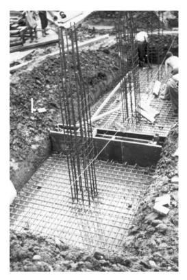
**Plate 15a.** Column base excavations are always liable to fill with rainwater. A sump should have been excavated beside each to permit dewatering before concreting
