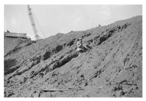
**Plate 7a.** Erosion of a newly placed embankment by rainfall runoff from the formation above. This is likely to be a contractor's risk, as it is 'a condition due to weather conditions' under ICE conditions Clause 12
