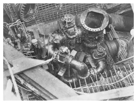
**Plate 11a.** An early photo of congested pipework being built in the base of a shaft, taking more than a week to complete. Hard hats must now be worn.
