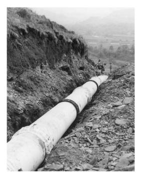
**Plate 6a.** A problem for the designer under the Construction (Design and Management) Regulations 1994 who has to pay 'adequate regard to the need to avoid foreseeable risks' (see p. 107 *et seq.*). The designer may decide a stable berm should be cut into the hillside before the pipe trench is excavated
