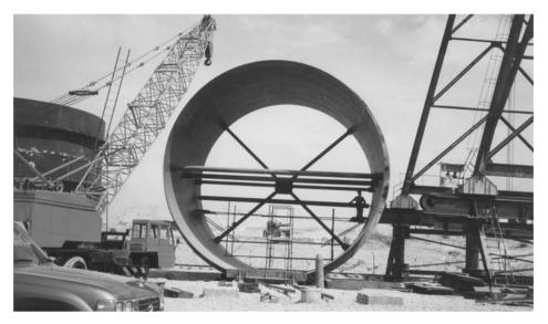
**Plate 5a.** Ten metre diameter steel can to form hydropower penstock, Ghazi Barotha Hydropower project, Pakistan 2001
