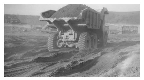
Plate 4b. A badly rutted formation, probably due to excessive moisture content of the fill
