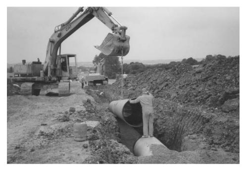
Plate 10a. It is almost universal to use the hydraulic excavator also as a crane
