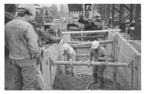
**Plate 12a.** On any job not properly supervised the strangest things can happen. It looks as if someone forgot the reinforcement until after the first placement of concrete. A resident engineer would stop the work and require it to be redone properly
