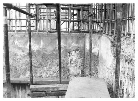
**Plate 16c.** Concrete which needs to be cut out: honeycombing and apparently inadequate cover to reinforcement
