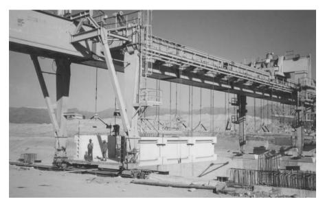
**Plate 11b.** A sophisticated gantry for handling and placing pre-cast concrete bridge and other units. Ghazi Barotha Hydropower project, Pakistan 2001
