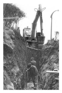
**Plate 7b.** An early photo showing unsafe conditions not now permissible. The designer would now have to consider any safer alternative route for the trench, or require a safe berm to be cut into the hillside first to give a shallower trench. The contractor must fully support the trench sides and require his men to wear hard hats.
