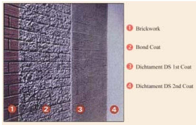
Waterproofing by Mineral Based Polymer Modified Coatings.
