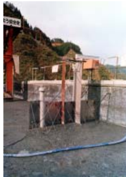
Figure 9. Installation of Water-stop and Drainage
