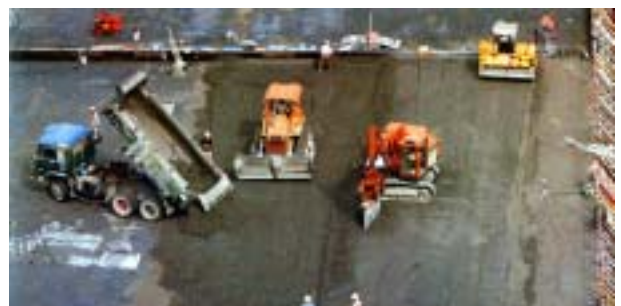
Figure 6. RCD Construction Method
