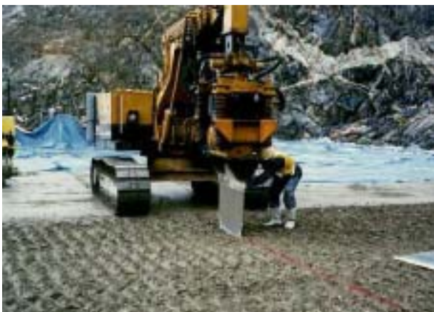
Figure 8. Installation of Transverse Joint
