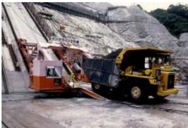
Figure 19 Dump Truck Mounted Incline
