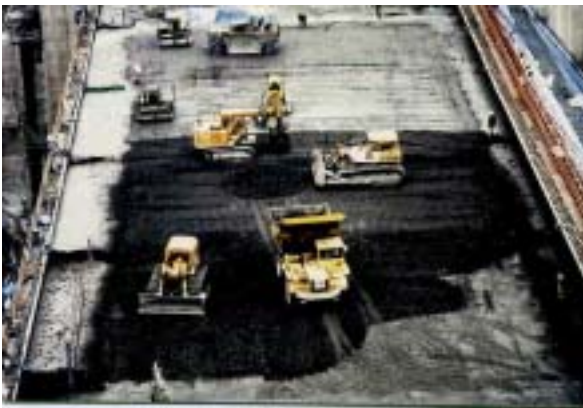
Figure 11. RCD Construction Method
