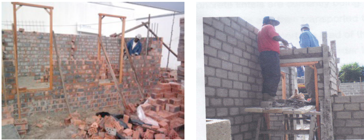
Figure 50: Brickwall and Lintel Construction
