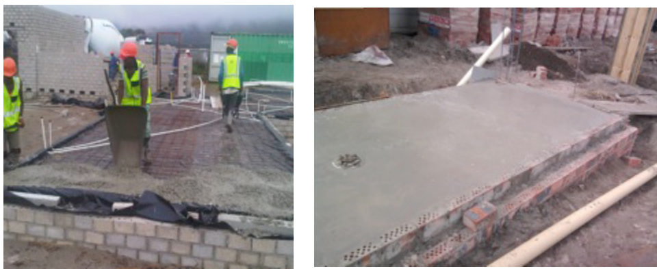
Figure 49: Production of the oversite concrete/surface bed
