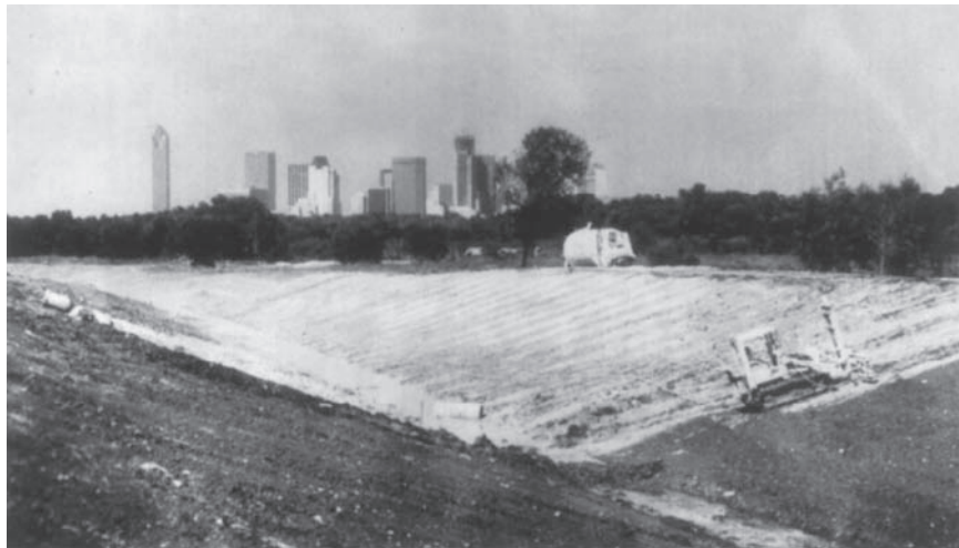
Figure 13.23 Slope stabilization of a canal bank by pressure injection of lime–fly-ash slurry (Courtesy of Hayward Baker Inc., Odenton, Maryland.)
