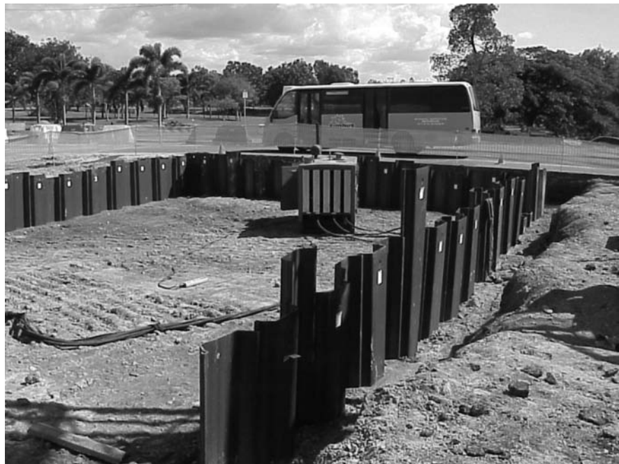
Figure 9.4 A steel sheet pile wall (Courtesy of N. Sivakugan, James Cook University, Australia)
