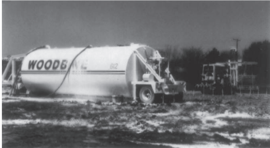
Figure 13.22 Pressure injection of lime slurry for a building pad (Courtesy of Hayward Baker Inc., Odenton, Maryland.)
