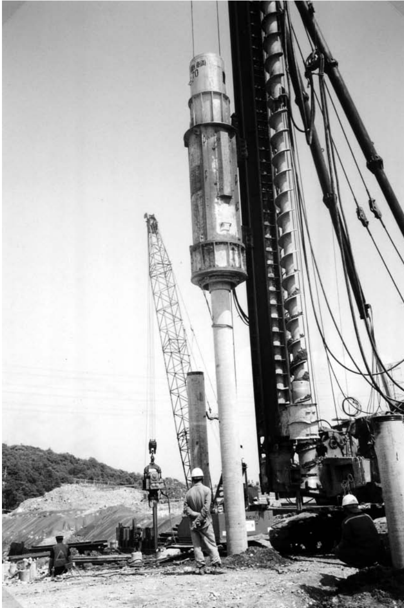
Figure 11.8 A pile-driving operation in the field (Courtesy of E. C. Shin, University of Incheon, Korea)
