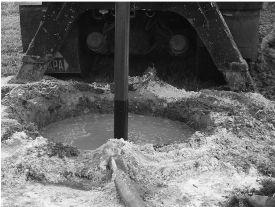
Figure 12.6 Drilled shaft construction using wet method (Courtesy of Khaled Sobhan, Florida Atlantic University, Boca Raton, Florida)
