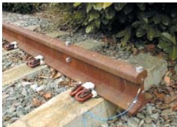
IRS-T 40 special grade cement was originally made for manufacturing concrete sleeper for railway line.
