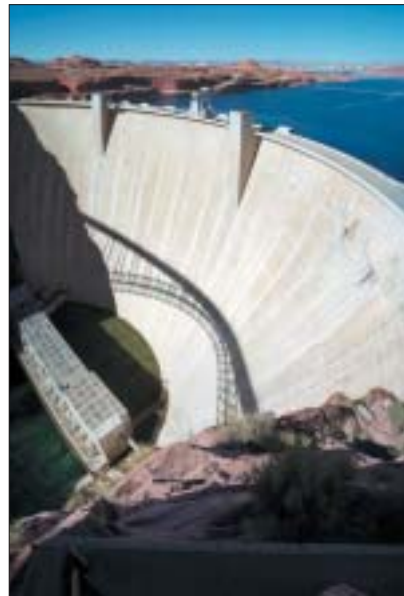
Low heat cement is made use of in construction of massive dams.
