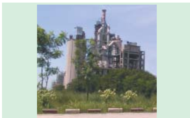
Part view of Cement Factory
